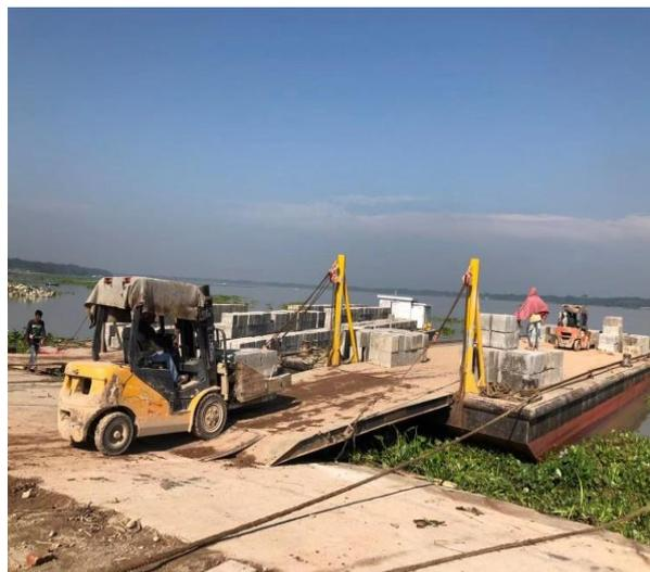
Figure 3-65: Loading CC Block on the berge in Polder 39-2C
