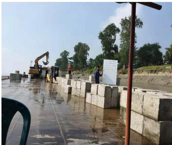
Figure 3-58: Dumping work in Polder-41/1
