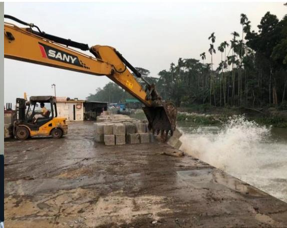
Figure 3-57: Dumping CC Block for river bank protection work (KM51+041-53+418) in Polder 39-2C
