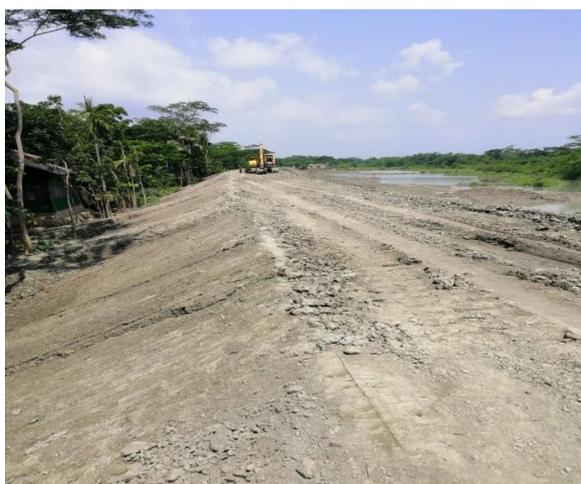
Figure 3-60: Earth Work for Embankment KM1+000 to Km2+000 in Polder 43 /2C
