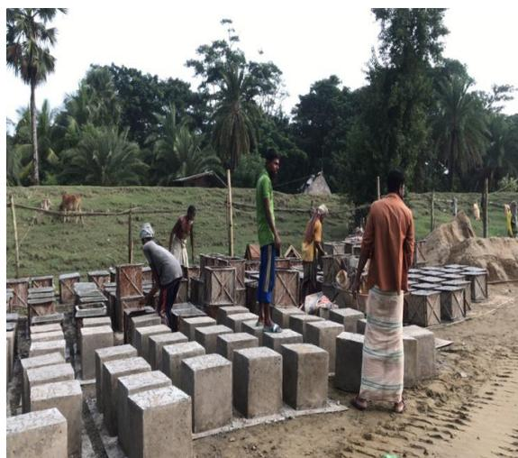
Figure 3-63: CC block manufacturing in Polder 47/2 at yard-1
